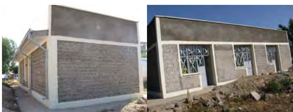
Front, Side and Rear View of the Constructed YFC
